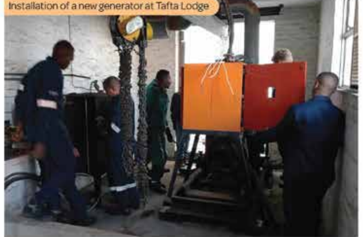
Installation of a new generator at Tafta Lodge
