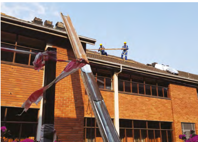
Robert Storm House roof and gutter replacement.
